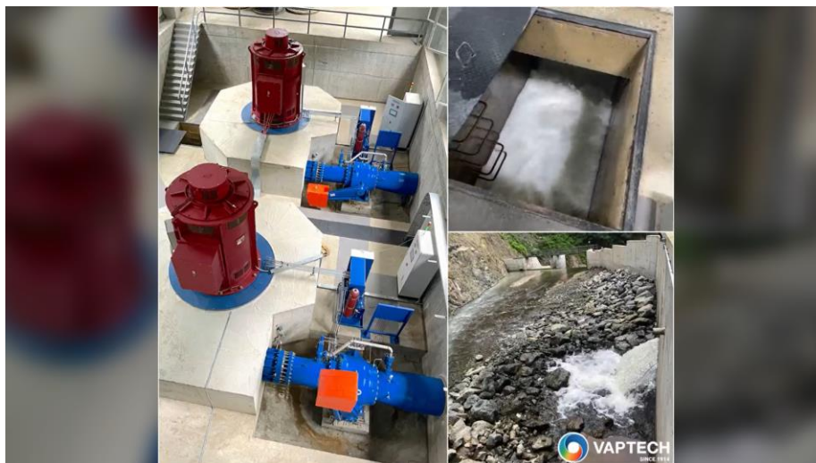
Hydropower plant developed with Vaptech technology and systems
